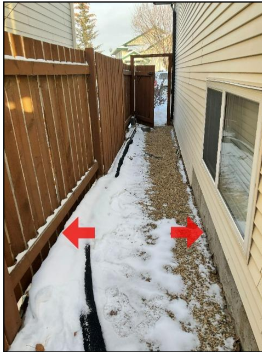
4. Discharge too close to building
